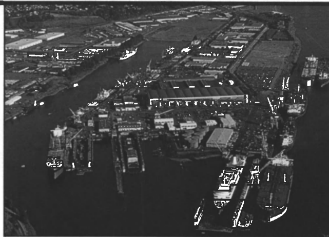
One of the largest, most complete ship repair facilities in the world, conveniently located on the US West Coast.
