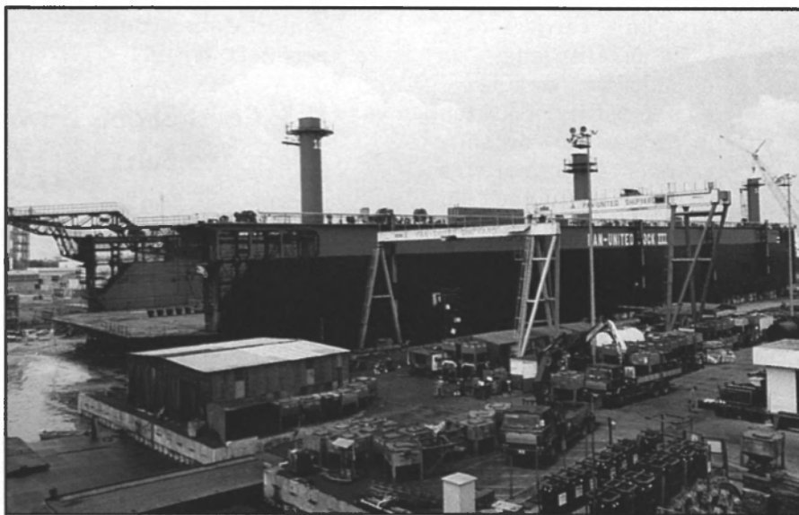
Pictured is the new 16,000-ton lifting capacity floating dock at Pan United Shipyard. The floating dock measures 615 x 120-ft. (187.5 x 36.5-m), and is able to dock vessels up to 50,000 dwt.
